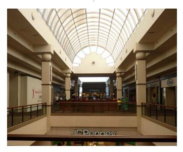
Problem: The existing 26-ft. x 120-ft. acrylic barrel vault skylight had failed and was beginning to leak, which created a life safety liability for shoppers. The intense glare and poor light diffusion also created an unpleasant visual environment for mall-goers and tenants alike.
