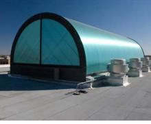
Problem: Existing glass skylight had deteriorated and was plagued by water leaks at the horizontal joints.
