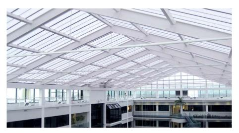
**Problem:** The 19,000 sq. ft. ridge skylight over the main atrium was severely discolored and deteriorating, resulting in a dark and dingy workspace.
