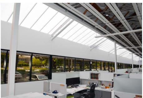
CPI replaced 9,000 sq. ft. of fiberglass skylight running the perimeter of the office building, that had yellowed and was leaking beyond repair.
