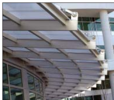
ID 27111 – Siemens Corporation Cafe, Cary, NC LiteBrow® Suspended Translucent Canopy & Sun Shade Architect: Hager Smith Design
