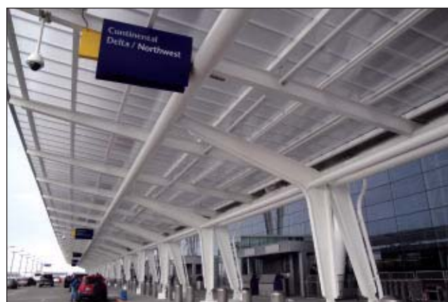
ID 20478 – Indianapolis International Airport, Indianapolis, IN Translucent 22,000 SF Single Slope skin-system dropoff canopy Architect: Domain Architects
