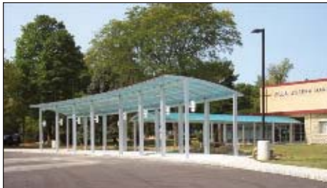
#20637 Villa Joseph Marie School - Model CRP custom walkway and drop off canopy
